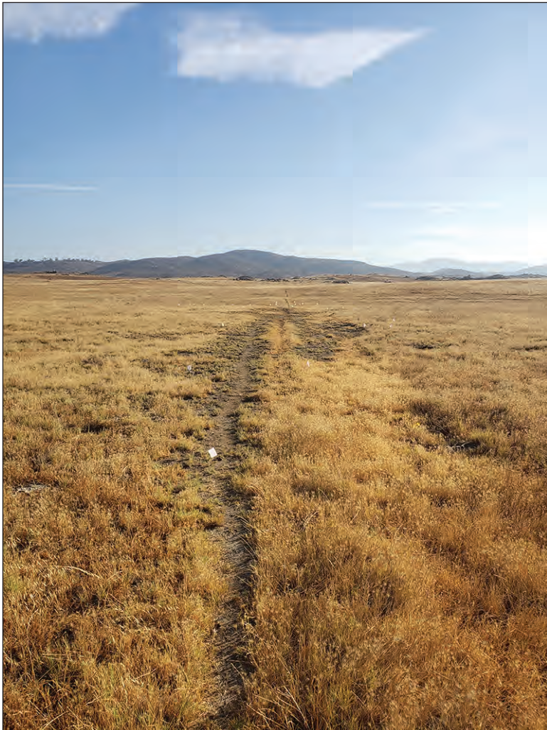
PHOTOGRAPH 25: View of RAAP17 before maintenance, taken July 13, 2022.
