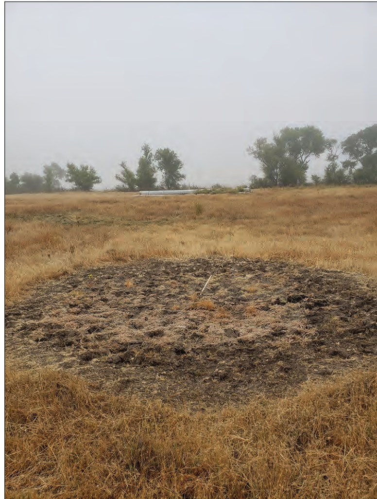
PHOTOGRAPH 18: View of EV3 after maintenance, taken July 12, 2022.
