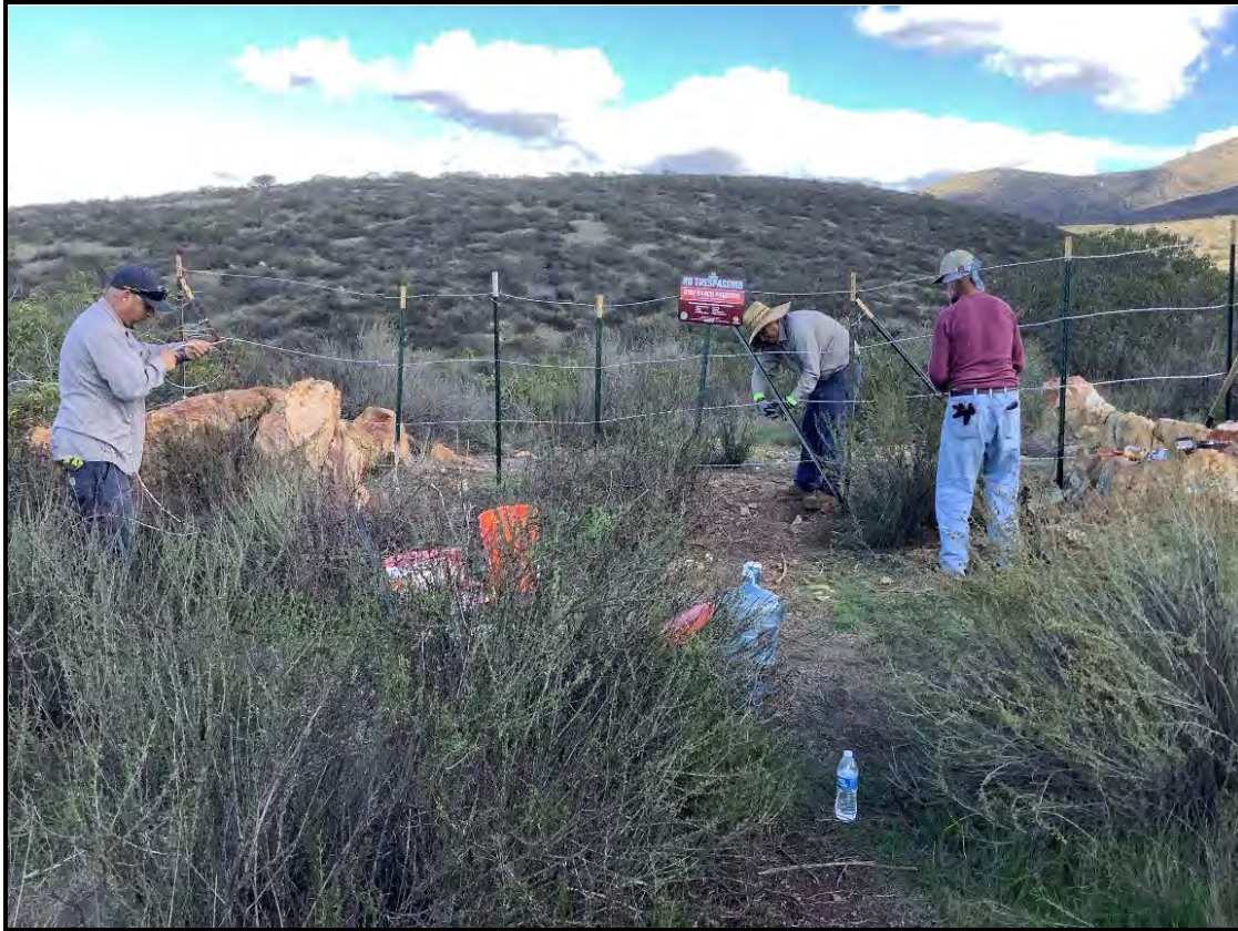
PHOTOGRAPH 29 RECON Crew Repairing Fence, Jamul Mountains Parcels, December 5, 2022
