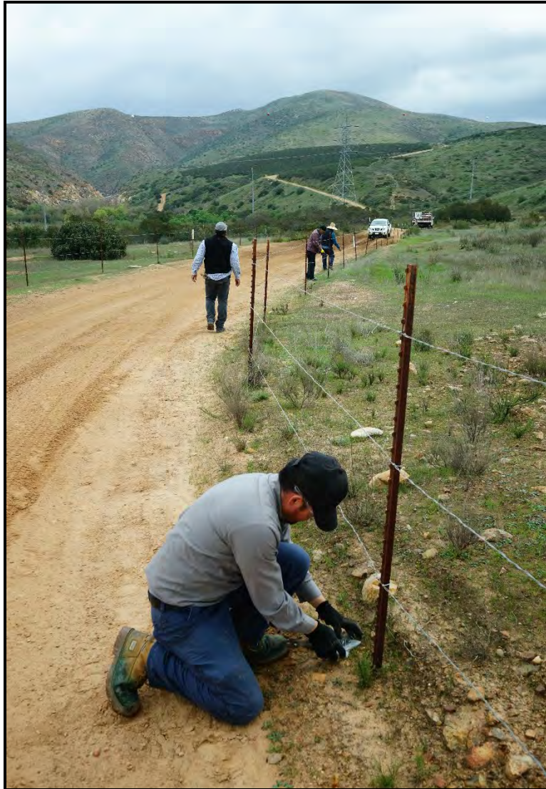
PHOTOGRAPH 30 RECON Crew Repairing Fence, Salt Creek Parcels, February 22, 2022
