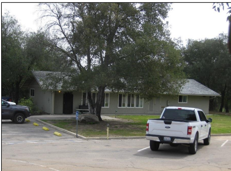
Figure 34. Fire Station Complex Main Building
