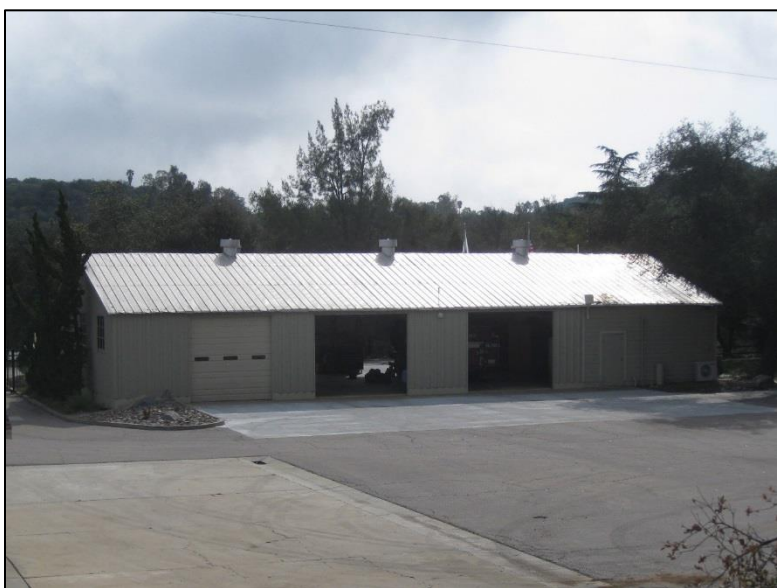
Figure 35. Fire Station Complex Garage
