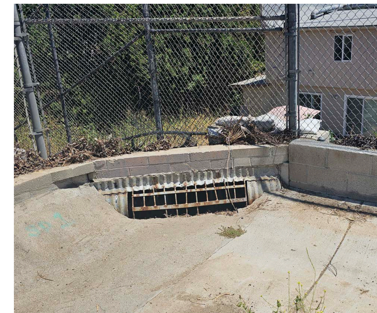
7 - Storm Drain Inlet
