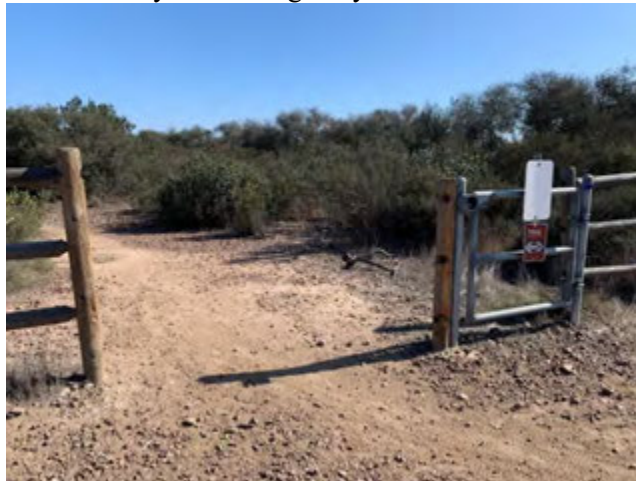
Figure 3. Wood fence vandalized at Del Mar Mesa, using a sawzall on the posts and beams, and a razor to deface the keep-out sign (white). This is also excessive use.
